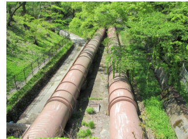
Some water is channeled through water-pressure pipes to the power generation station.
